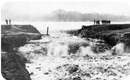
Opening the Montlake Cut, August 25, 1916. Over the course of three months, Lake Washington water was slowly released into the cut past gates at the other end, lowering the big lake by 9 feet to create the ship canal. The lake's shoreline was forever changed. (Richard McDonald Collection)
